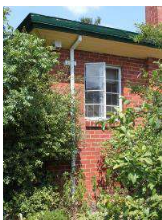
Old rectory exterior. Note the gutters are behind the fascia boards. Photo PG
