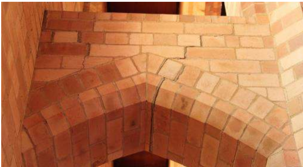
Cracks in cross arches. Photo: PG 2015
